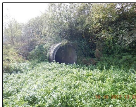
B) Surface water drain outlet, looking south
