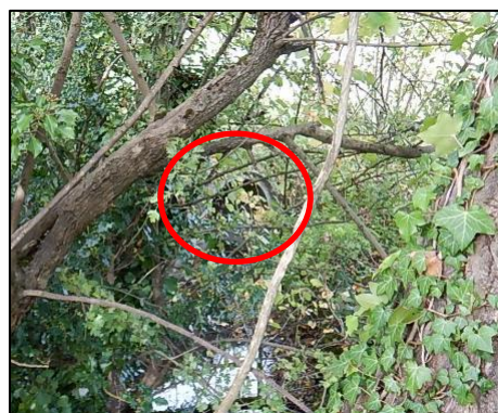
D) Inlet for OPW drainage channel (red circle)
